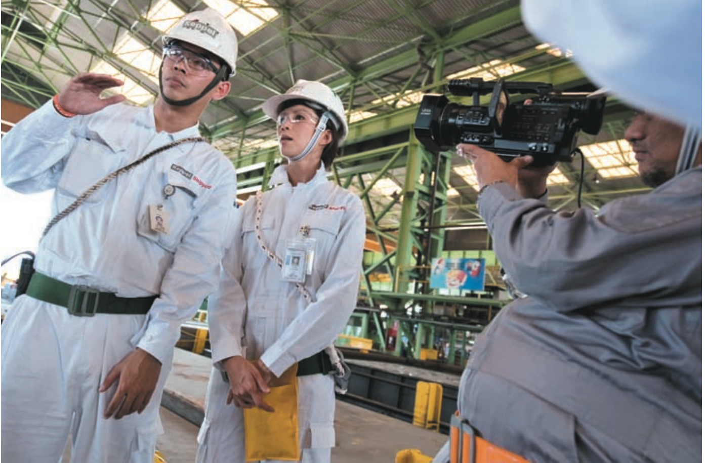
Terry Wong, Project Manager of the FPSO, P-57, shows Wong Lilin around the hull workshop where steel is being cut for the renewal of the hull's bottom plate
