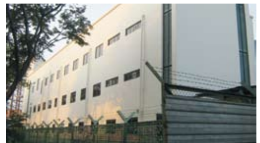
New building at 15 Benoi road
