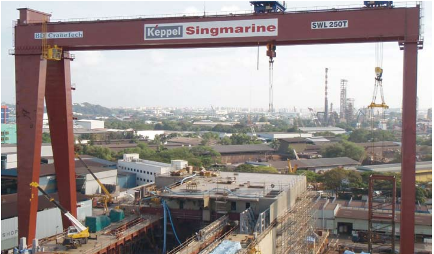
Block erection using the newly installed 250 tonne gantry crane
