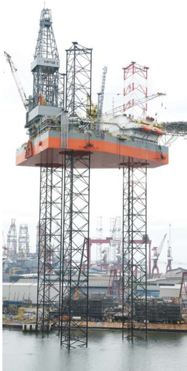
VIRTUE I is the second jackup rig Keppel FELS has completed for Jindal
