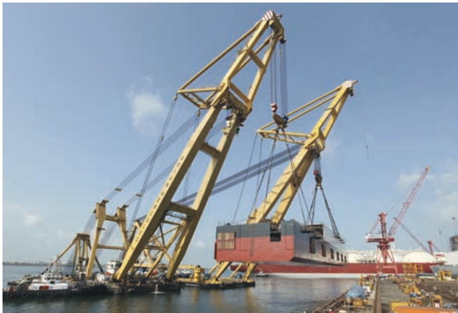
Lifting the strips of the derrick lay barge requires careful coordination
