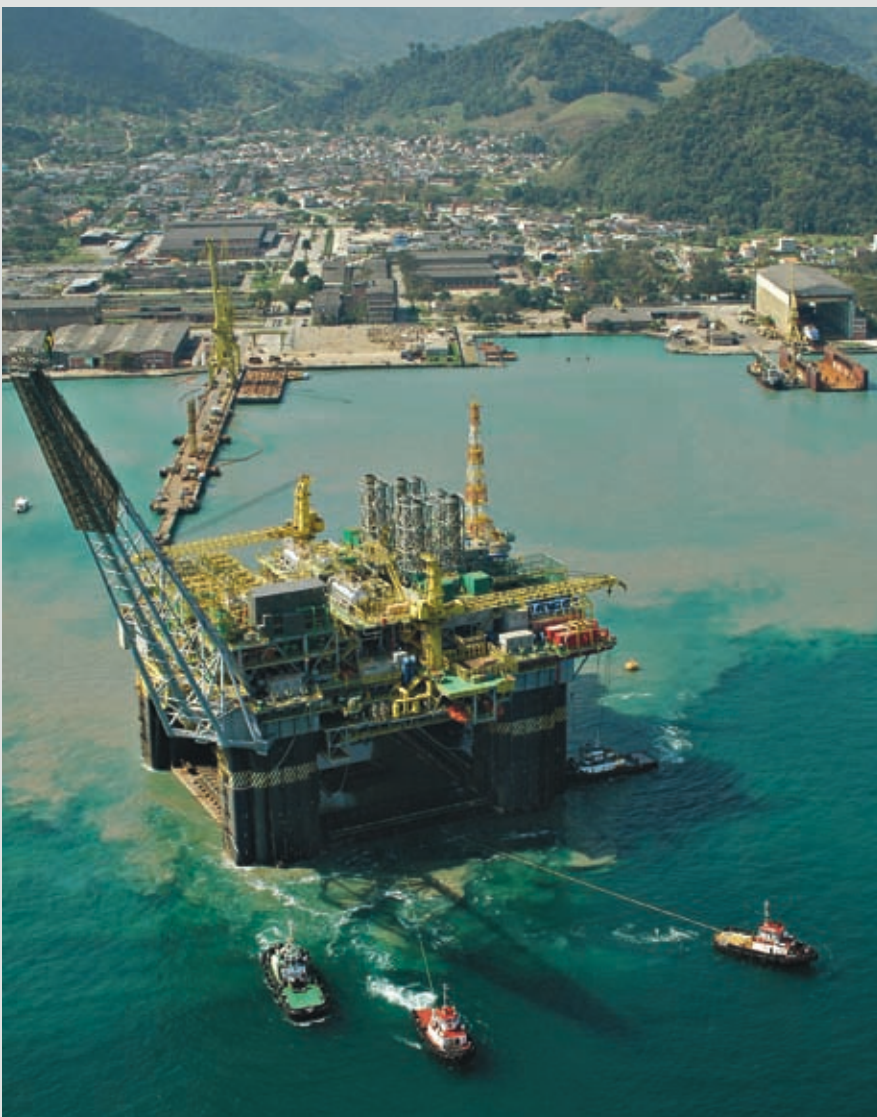
Keppel O&M continues to achieve many 'firsts' through its BrasFELS shipyard, such as the completion of FPU P-52 (above) and P-51 for Petrobras
