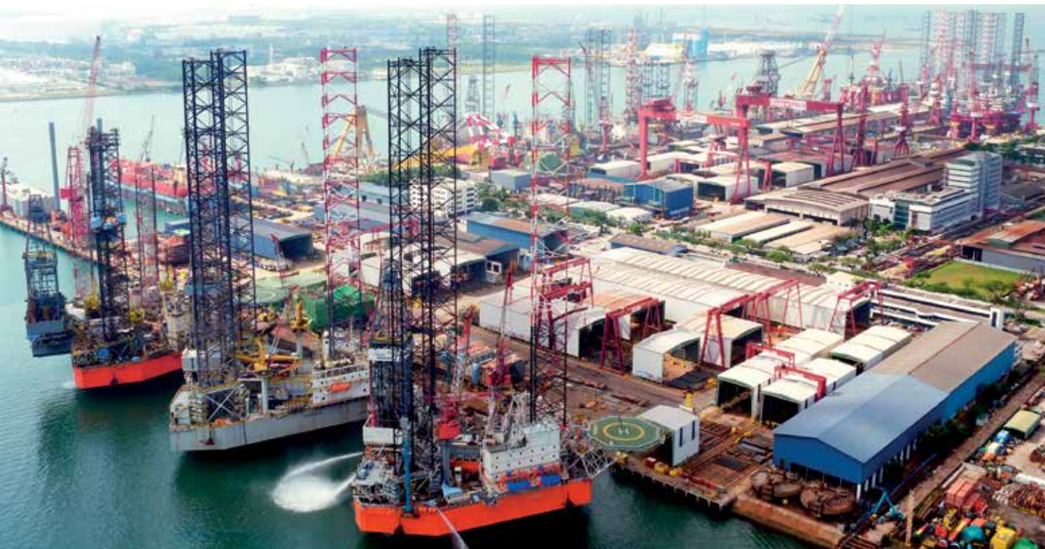
Keppel O&M continues to keep busy with its backlog of orders as well as repair, upgrade and modification projects
