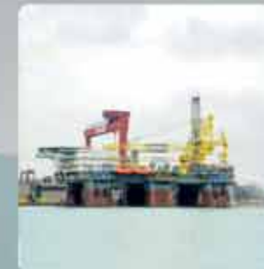
11 PV Drilling V
