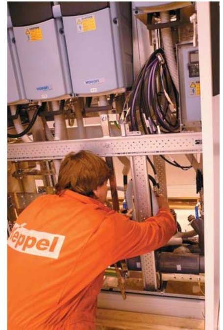
Busy at work on the power systems
