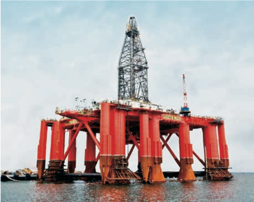
Strong teamwork and camaraderie enabled the teams from Stena Drilling and Keppel FELS to return Stena Clyde to mint condition
