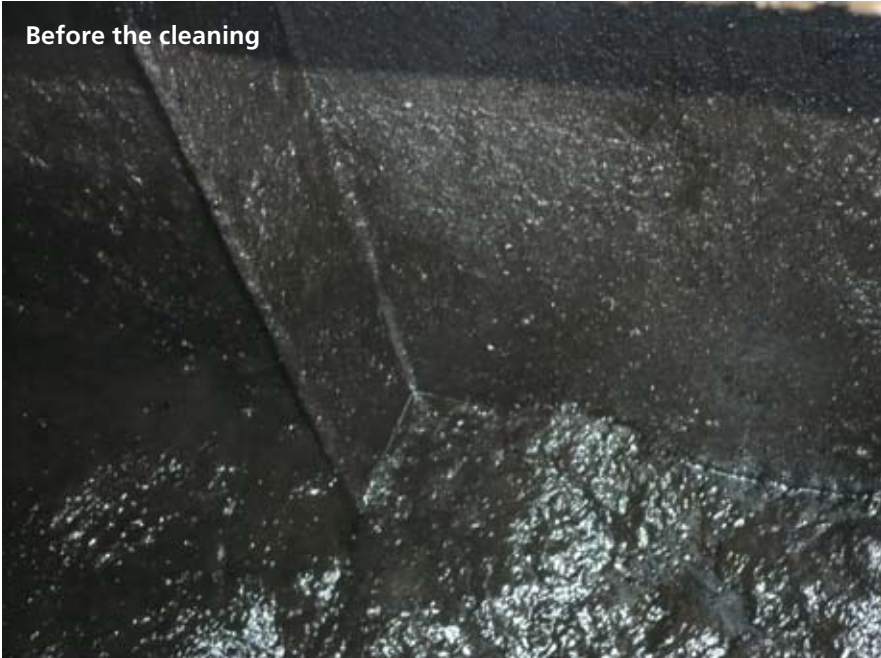
Close-up pictures of the tank surface conditions before and after cleaning using Bio-OSR
